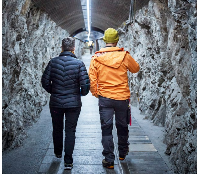
The trip back down to the valley first leads through solid rock – a reinforced tunnel connects the research station with the summit stop of the Jungfrauoch railway. Photos: Franziska Frutiger
